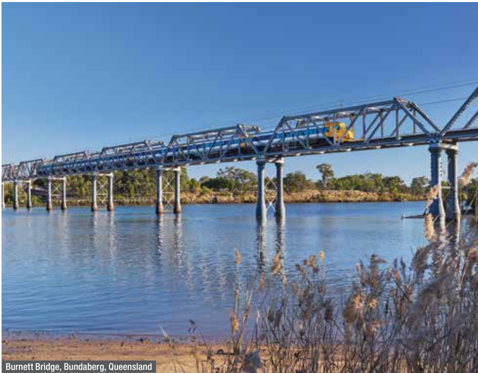
Burnett Bridge, Bundaberg, Queensland
